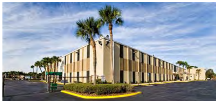
Jacksonville's Cologix, a colocation and disaster recovery provider, houses the DCA's Network Operations Center.
